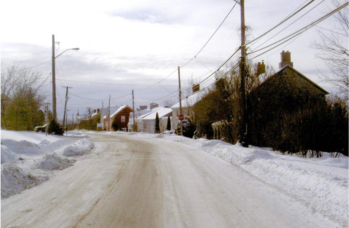
The same view today looking south down Main Street – the buildings along the right (west) side of Main Street are largely unchanged.
